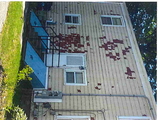
Condition of one of the houses
